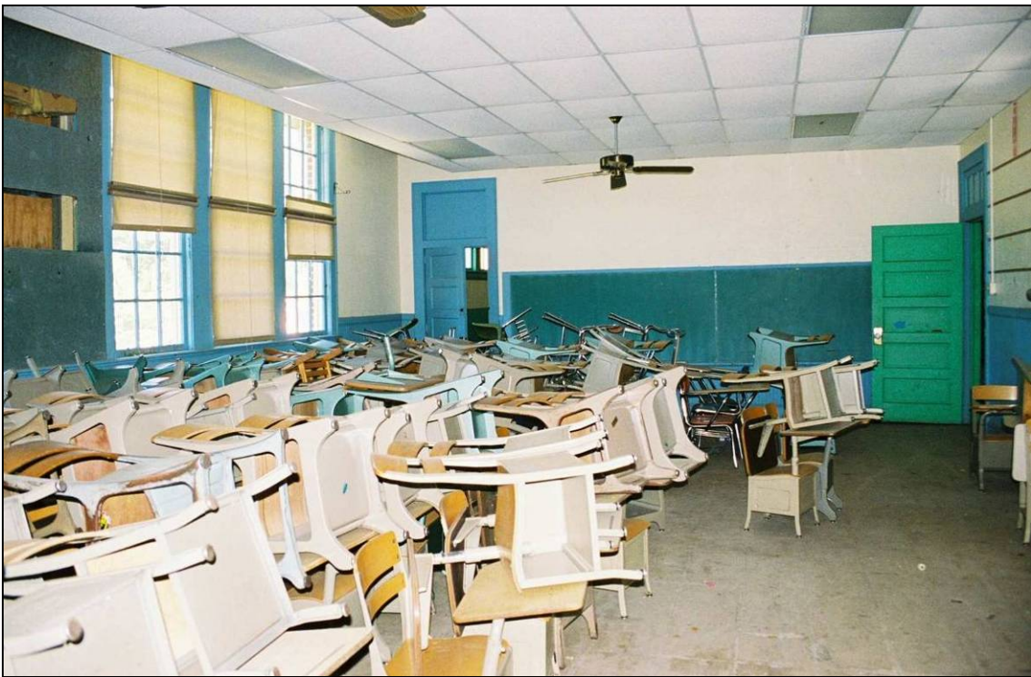
Plate 208. Spring Hope School: west central classroom; note original doors, transoms, and replaced blackboard
