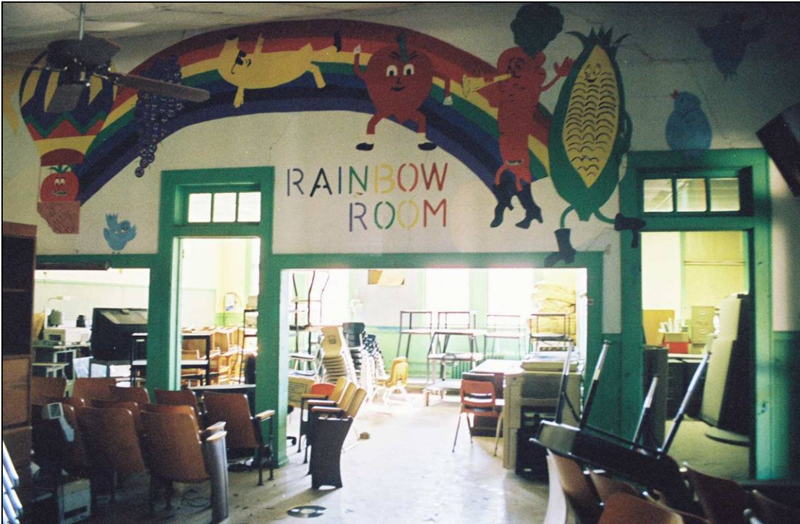
Plate 205. Spring Hope School: view from hyphen to east central classroom
