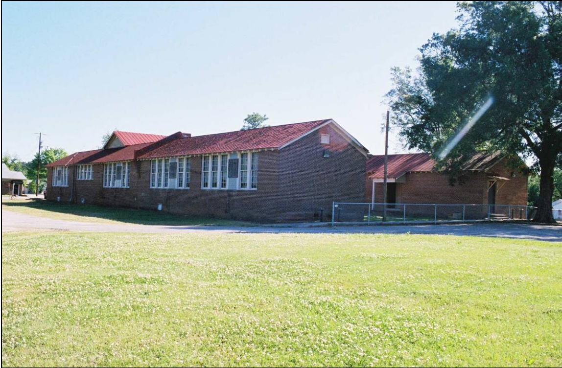
Plate 197. Spring Hope School: west side and south rear elevations with additional classrooms at center behind elevated firewall
