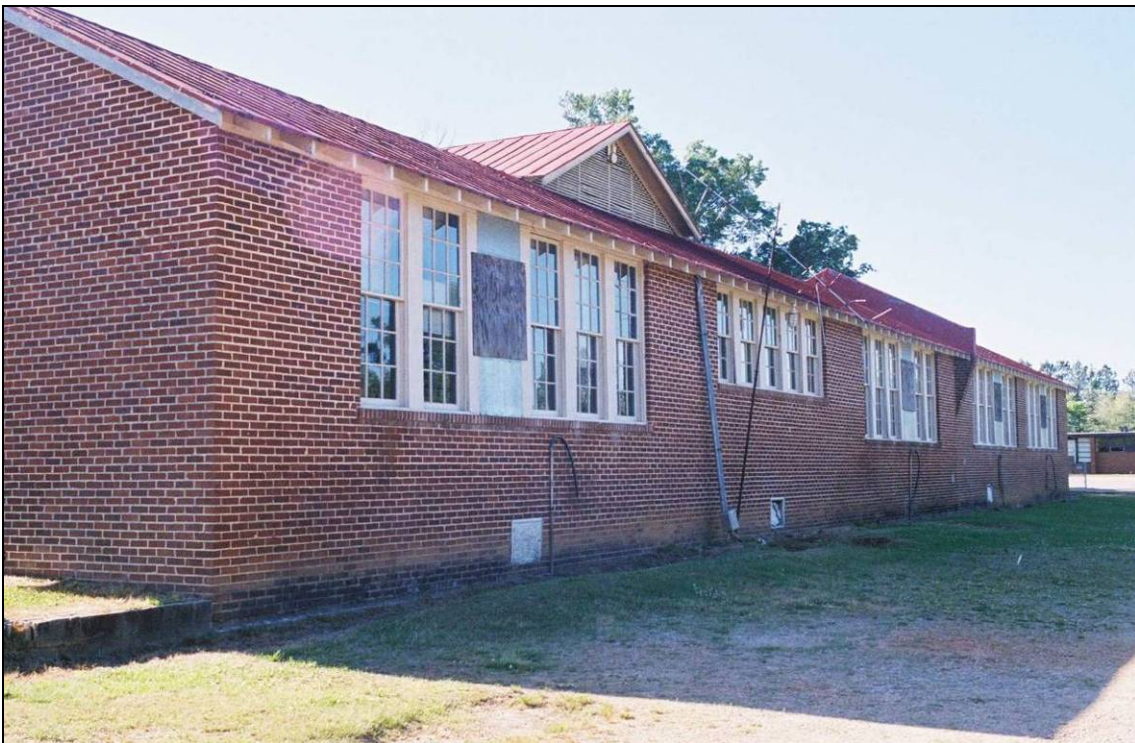
Plate 200. Spring Hope School: edge of north front and east side elevations; note shorter windows of industrial room and firewall raised between initial end of school and later addition
