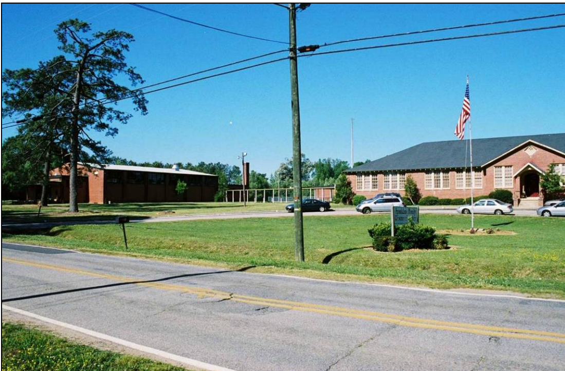
Plate 210. Spring Hope School: looking southwest from Pine Street at campus with 1941 high school building at right and 1950s buildings at center and left
