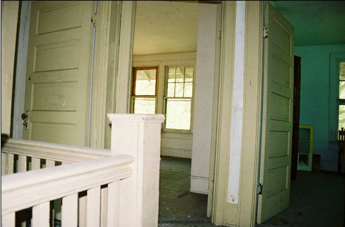
Plate 221. Spring Hope Teacherage: second floor hallway with entries to bedrooms; note intact cross-panel doors, surrounds, and stair newel and balusters
