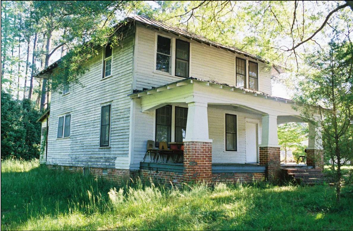
Plate 213. Spring Hope Teacherage: west side and south front elevations
