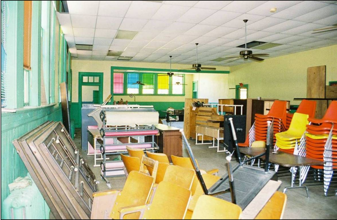
Plate 207. Spring Hope School: view from hyphen through removed partition to industrial room
